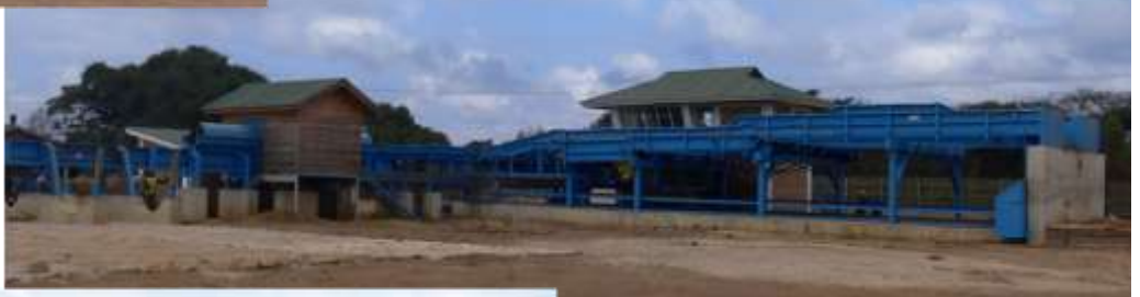
The intake to the log sorting line with the control room in the middle and the scanner to the left. A crane for offloading logs from the incoming trucks will be mounted at the very right, significantly reducing operation costs.
